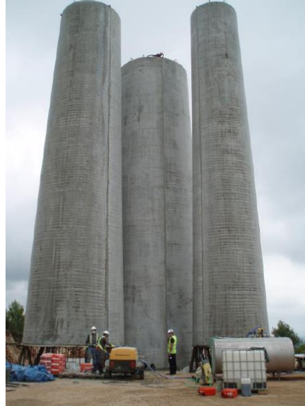
Figure 3-3 AW3000 concrete tower segments
