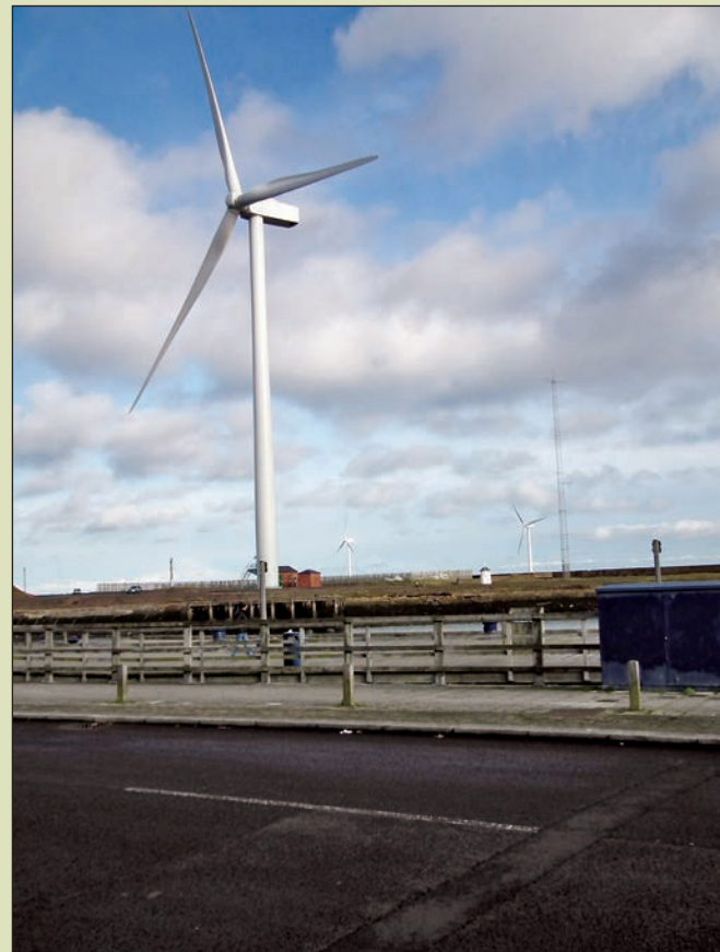
This 130m turbine on Blyth’s East Pier is one of the tallest built in England.
