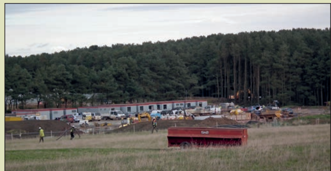
The wind farm construction base at Middlemoor near North Charlton.
